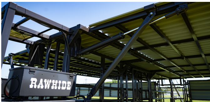
Roof with brace from outside
